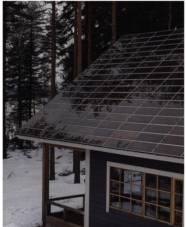
Figure 6.5 Roof reflects surroundings. private house, Laukaa (FIN); design: Soilikki Suntola, 1992
