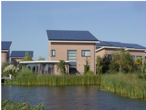
Figure 9.5 Multiple of panels define the size of the roof. The architect adjusted the rim and edges to create a clear surface. Mayersloot Langedijk. Design BEAR-iD, Tjerk Reijenga
