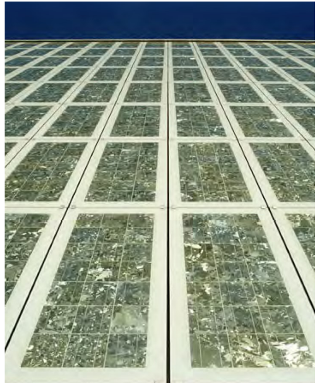
Figure 6.4 Prominent texture and green coloured cells define the architecture. Paul-Horn Arena, Tübingen, (BRD); design: Allman-Sattler-Wappner Architekten, 2004
